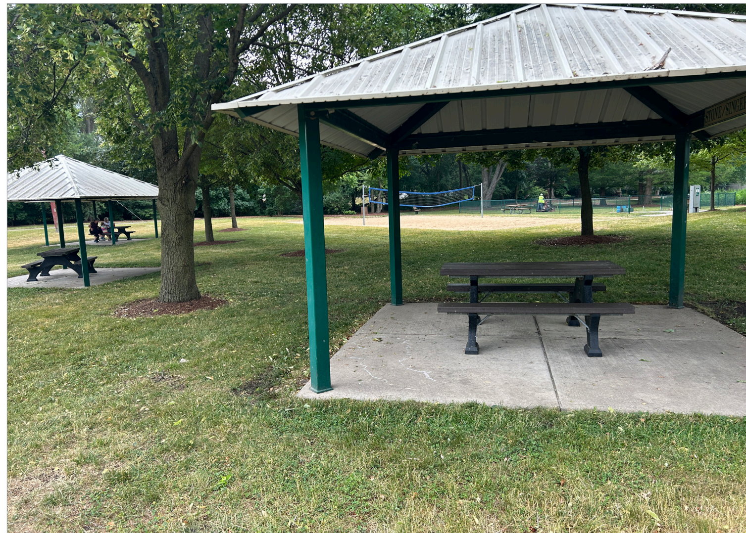
5. Shelter Renovations and Path Connections
